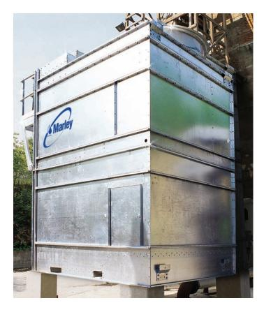
The AV Series has 38 factory assembled tower models with 117-390 nominal tons per cell.
